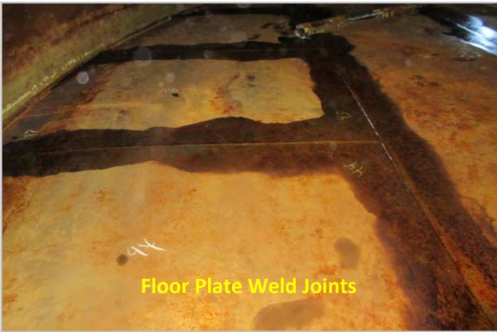
Floor Plate Weld Joints
