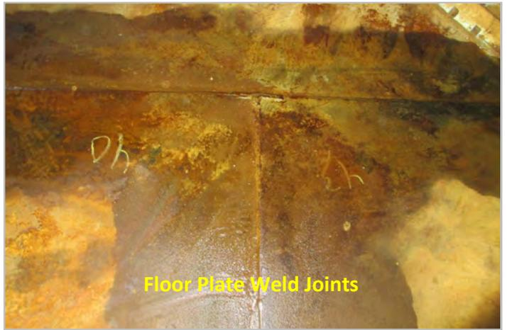
Floor Plate Weld Joints
